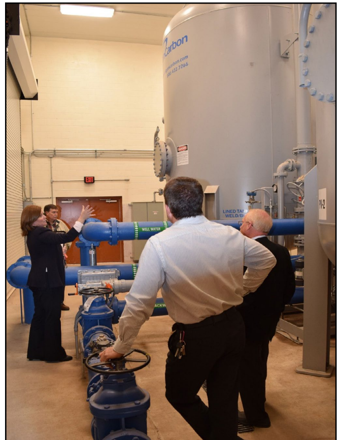
Horsham Township Council and Horsham Water & Sewer Authority tour a completed PFAS treatment filter on September 3, 2017.
