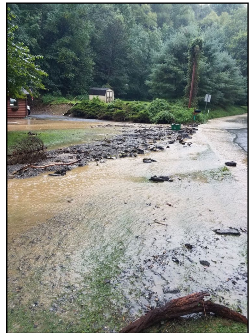
Flooding on Dark Hollow Road from Kreutz Creek during the 2018 event
