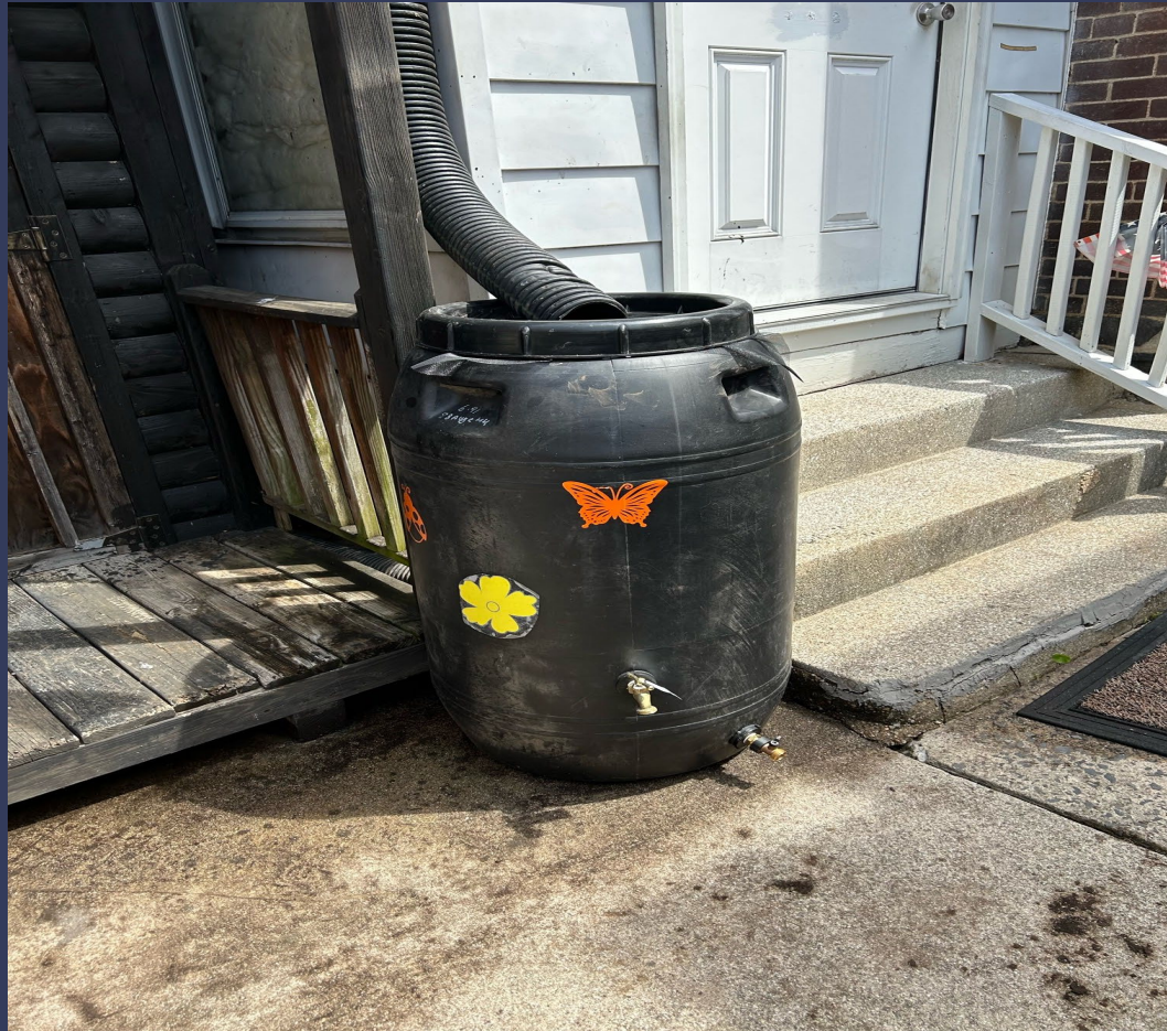
An extension pipe was added to the overflow to water the garden in the back yard.
