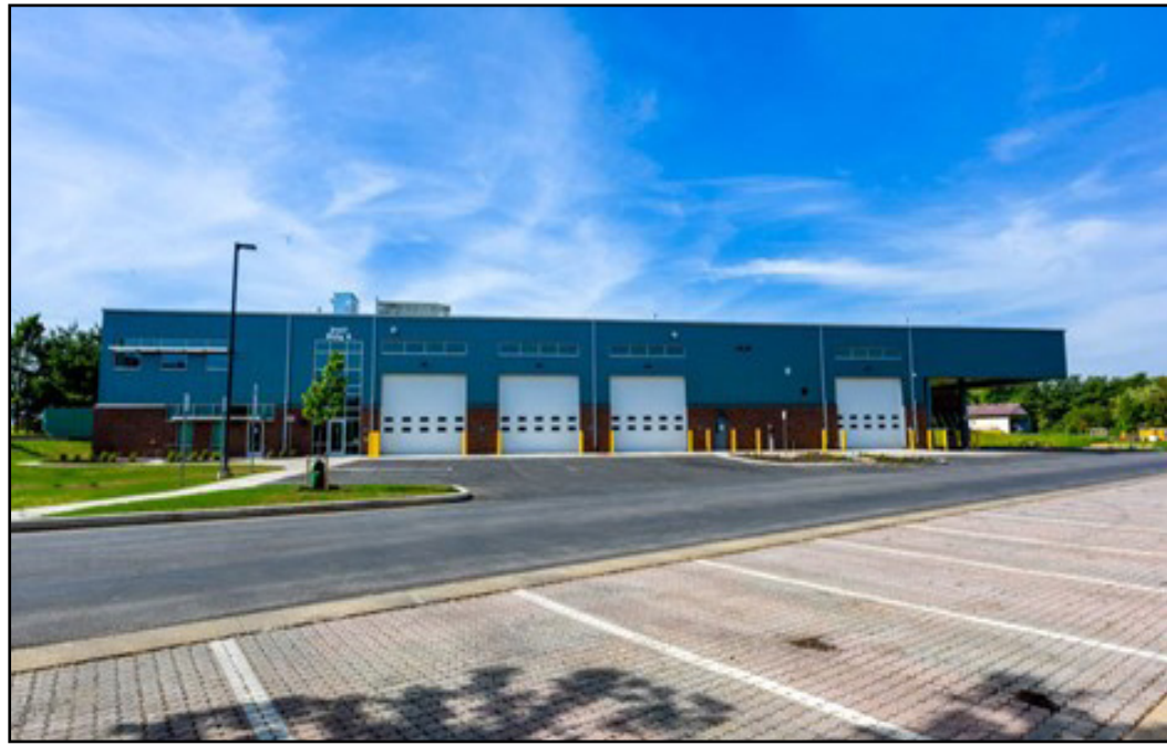
Ferguson Township LEED Gold Certified Public Works Building
