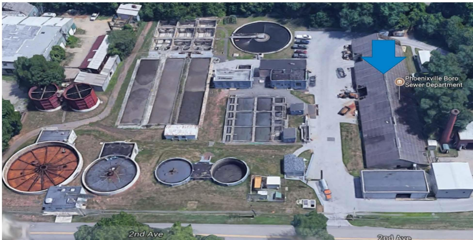
Borough of Phoenixville WWTP
