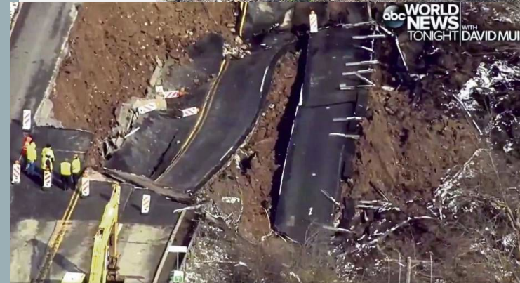
April 7, 2018 Landslide on Rte 30
