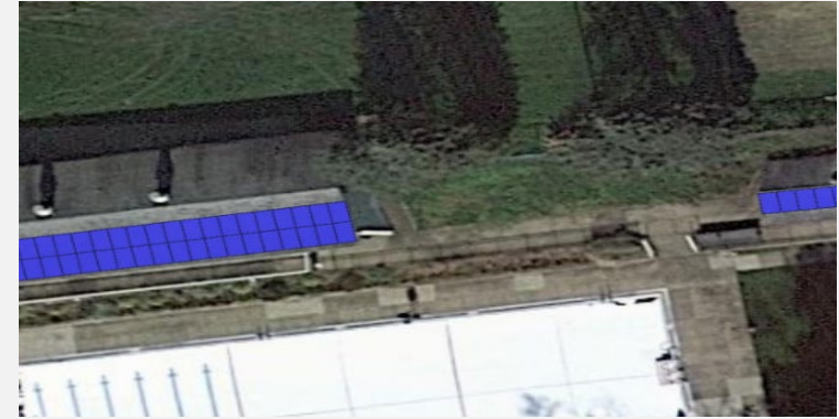
Siemens Industry, Inc. Community Pool
