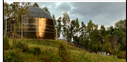
Baldwin Equalization Tank Baldwin Borough
