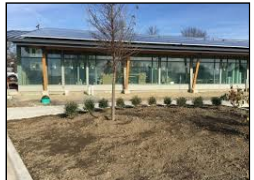
Forest Hills Municipal Building - Volpatt Construction - January 2018
